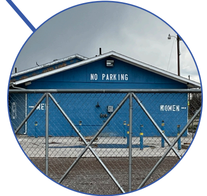
4. Unsanitary or Unsafe Conditions
