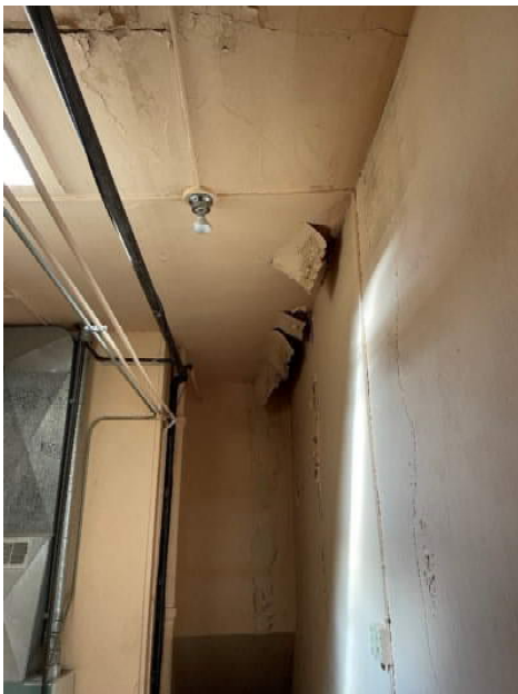
Photo 15 – Water damage to the second-floor ceiling (above the stair) at 215 W. Lincolnway.
