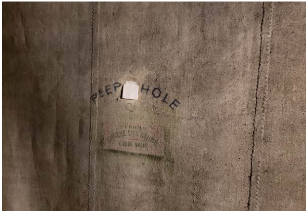
Reverse side of asbestos curtain at peep hole flap
