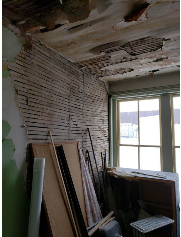
Ceiling and wall plaster water damage at rooms on South side
