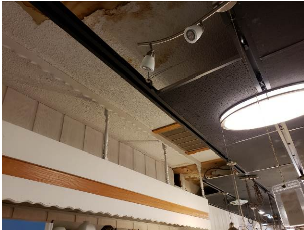
Tenant ceiling showing historic tin ceiling (north end)
