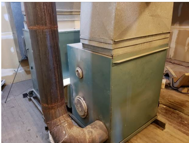
Furnace in Southeast room feeding First Floor lobby below
