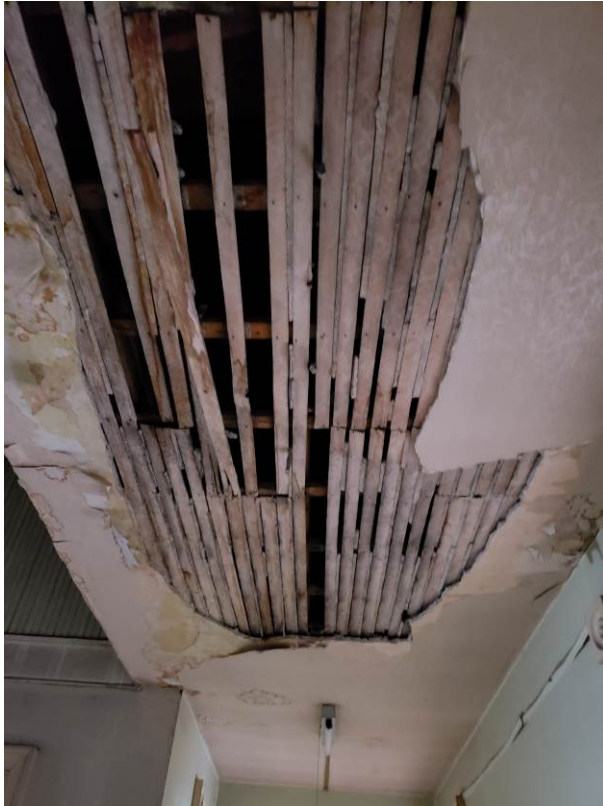
Ceiling plaster water damage
