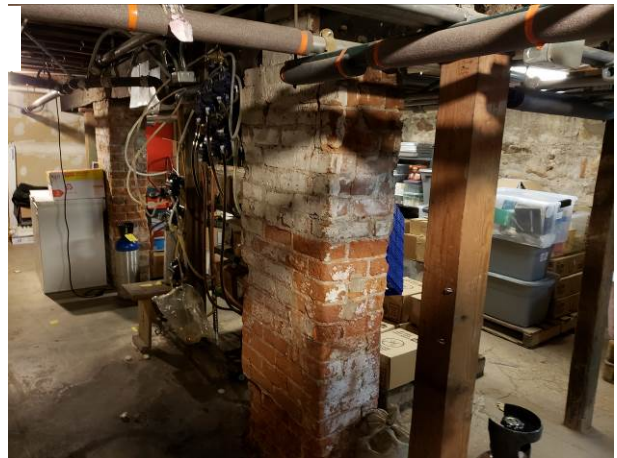
Masonry support column
