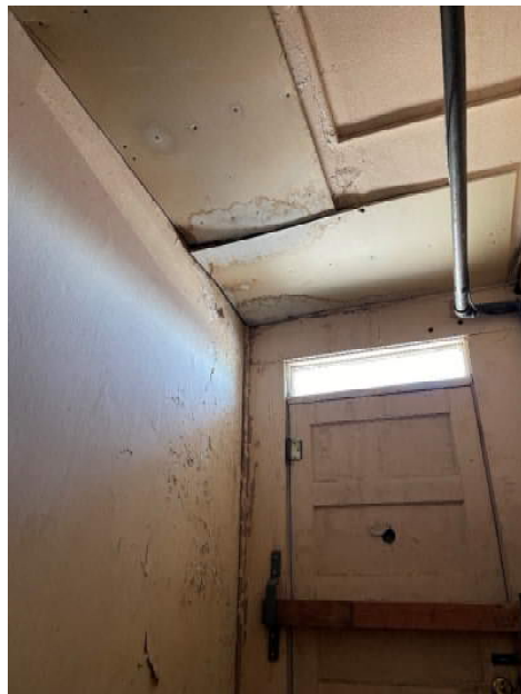
Photo 16 – Water damage to the second-floor ceiling (above the south door to the low roof) at 215 W. Lincolnway.
