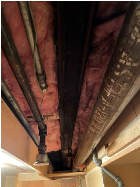
Photo 13 – Fire damage to the main floor joist as seen from the north end of the basement at 215 W. Lincolnway.
