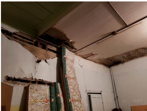
Water damage to plaster detail
