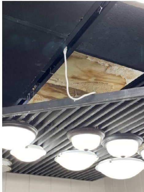
Photo 14 – Water damage to the main floor ceiling at 215 W. Lincolnway.
