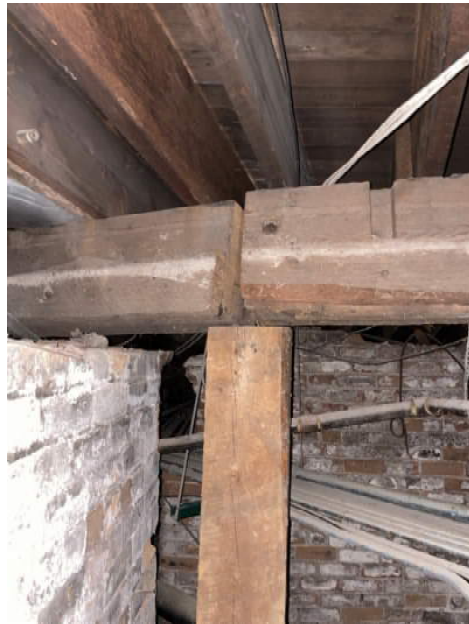
Photo 18 – Auditorium floor framing. Girders do not have solid bearing on post.
