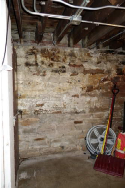
Photo 1 – General condition of stacked stone foundation wall. Efflorescence is visible in the top left corner of the wall.
