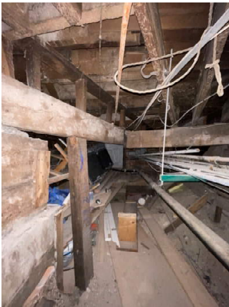
Photo 19 – Poor workmanship framing modifications under the Auditorium floor.
