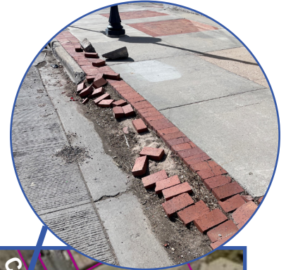
3. Deterioration of Site or Other Improvements
