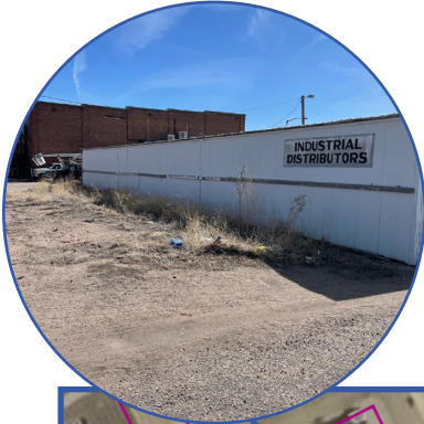
1. Deteriorated or Deteriorating Structures
