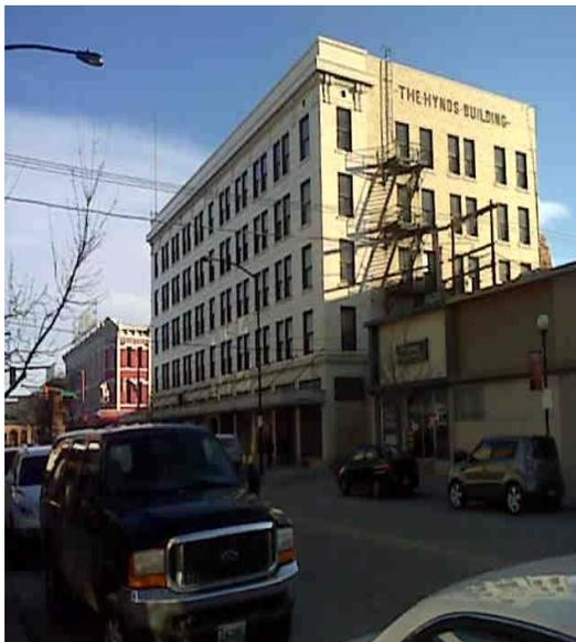
“The Hynds Building incorporated an enormously advanced design for its time. The structure has no interior or exterior supporting walls. Its mass is carried on a steel ‘T’ beam frame, with poured concrete ceilings and floors. In keeping with Mr. Hynds’ wish that the building be fireproof, no wood was used in its construction. All doors, casings, windows, and frames are metal, as is even the decorative picture rail.
