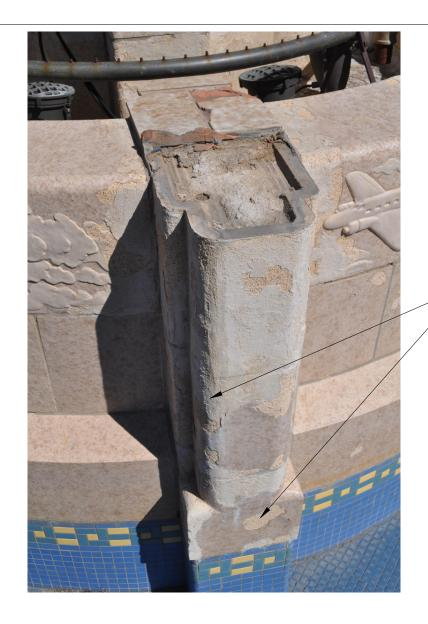
REMOVE PREVIOUSLY INSTALLED PATCH MATERIAL FROM JOINTS. REMOVE OR SMOOTH SURFACE OF DAMAGED TERRA COTTA TO BRING NEW SURFACE TO MATCH ADJACENT UNDAMAGED SURFACES
