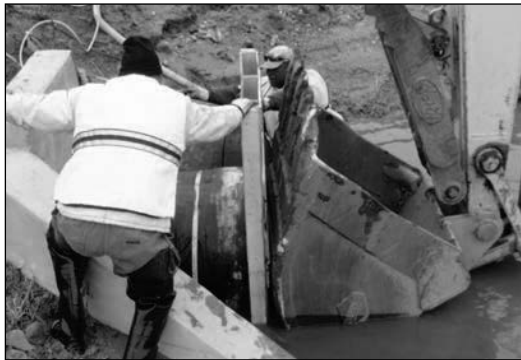
Pallet Push method for installing CheckMate® Valve
