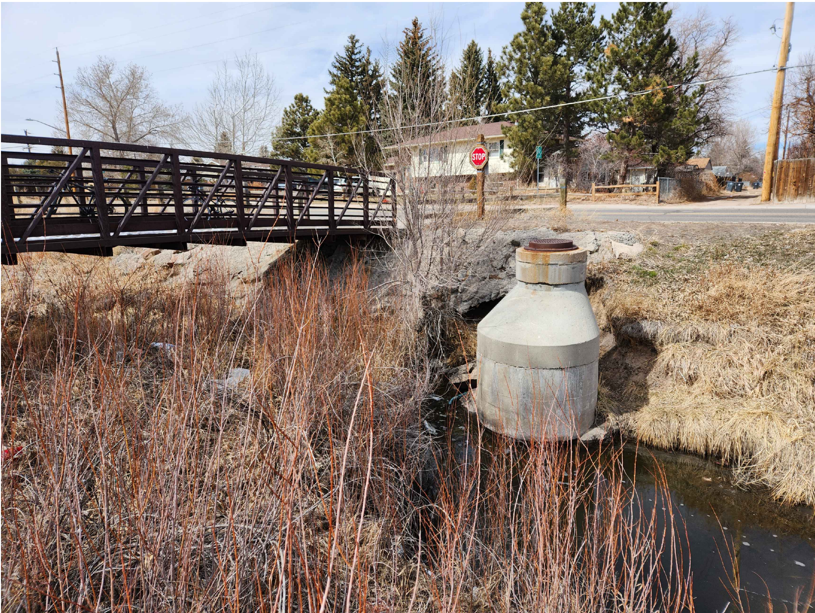
PHOTO 4: BANK EROSION AROUND SANITARY SEWER MANHOLE
