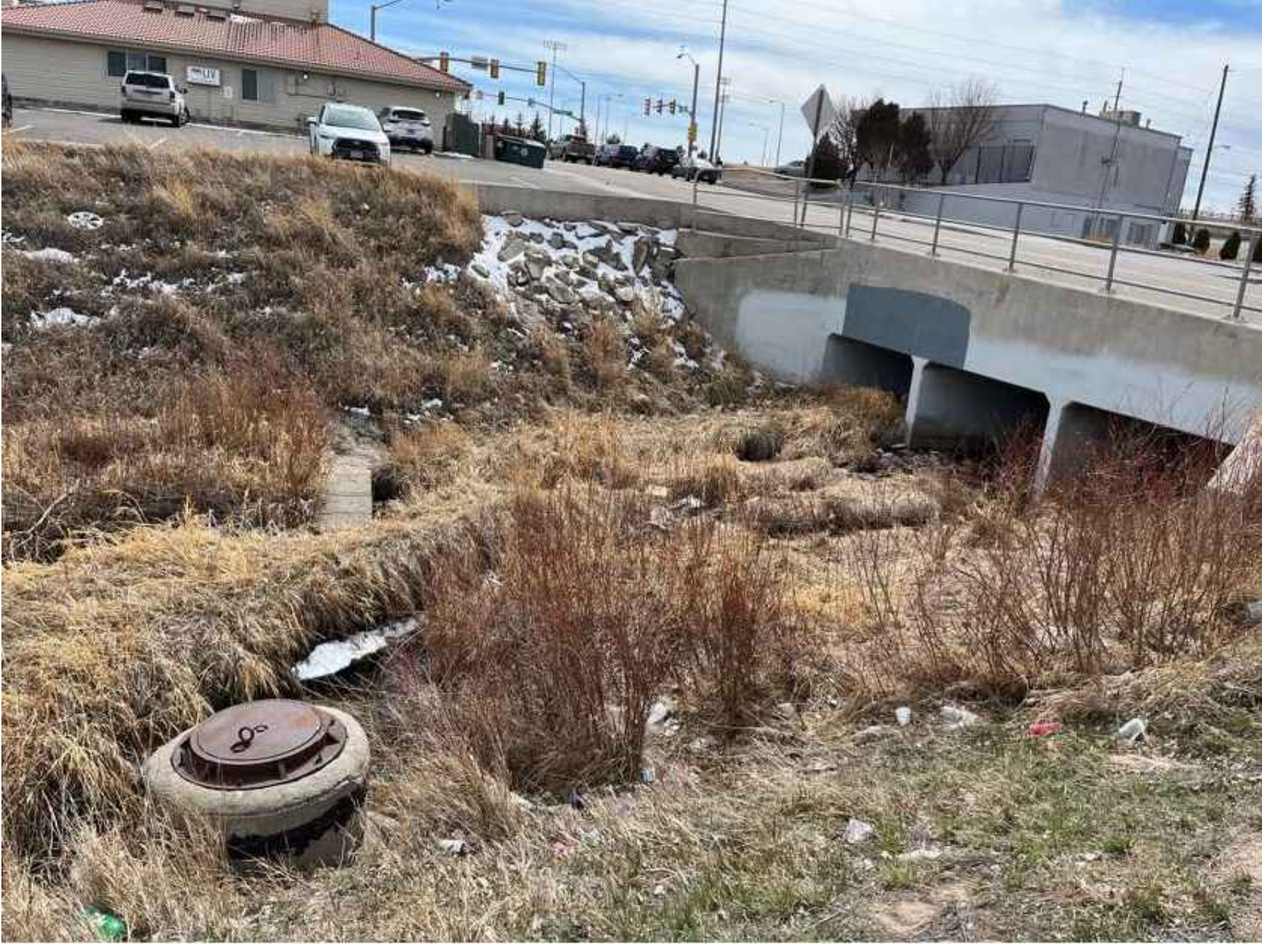
PHOTO 3: EXPOSED SANITARY SEWER MANHOLE
